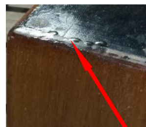
Dried drops of shellac on the bottom of the radio
