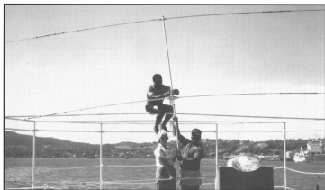
Installing the long range radio antenna on the ship's rear deck
